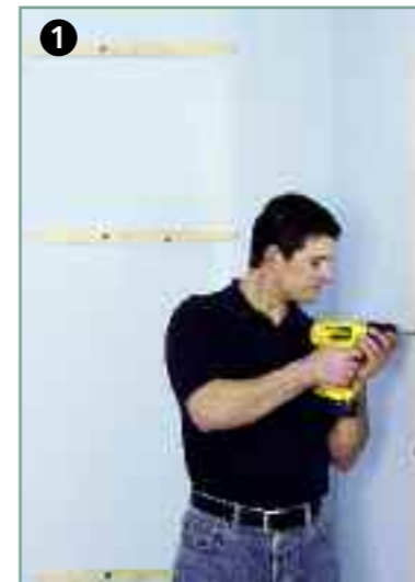
Position and fit the fixing batons to the wall.
