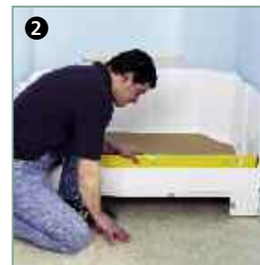
Locate, level and fix the base.
