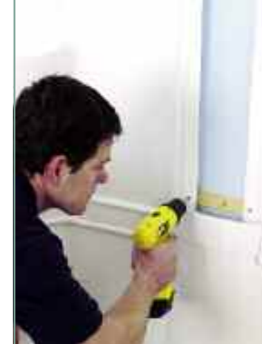
Slot the side panels to the base and fix to the back wall batons, using the spacer provided to ensure that the correct gap is left for the back panel.
