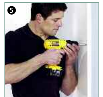
The front edges of the side panels can then be secured to the side wall batons and the fixing screws will be concealed by the door frame.
