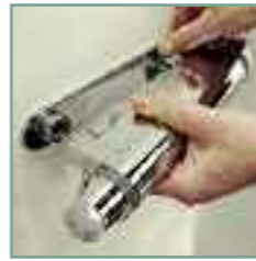
The mixer simply connects to the hot and cold feeds with the valve nuts.
