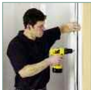
When fitting the shower door position the wall channels and drill the screw holes.
