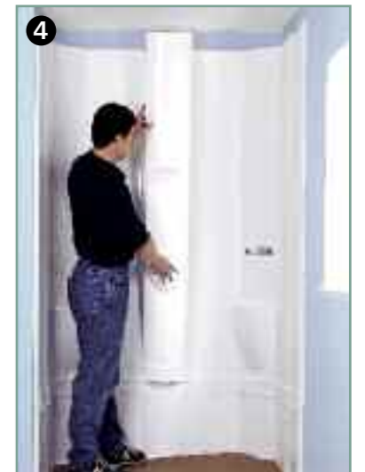
The back panel can then be slotted into position and secured with a single screw.
